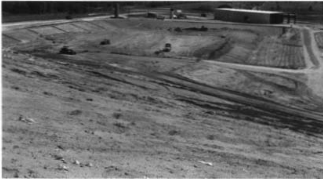
Figure 39. A new cell being prepared at the Marion County landfill, showing plastic liner on left and rear walls. The liner has been covered with sand on the other two walls for protection. Note the six leachate collection pipes on the left wall and the 30,000-gallon leachate holding tank in the left background (from Lane and Hoenstine, 1991).
