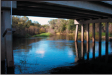
A bridge over the Econlockhatchee River (USF)
