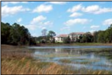
Some of the apartments being built on the western side of the lake in January 2002 (USF)
