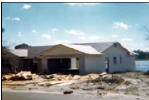
Marchetta's house in early construction (Heckenbach)
