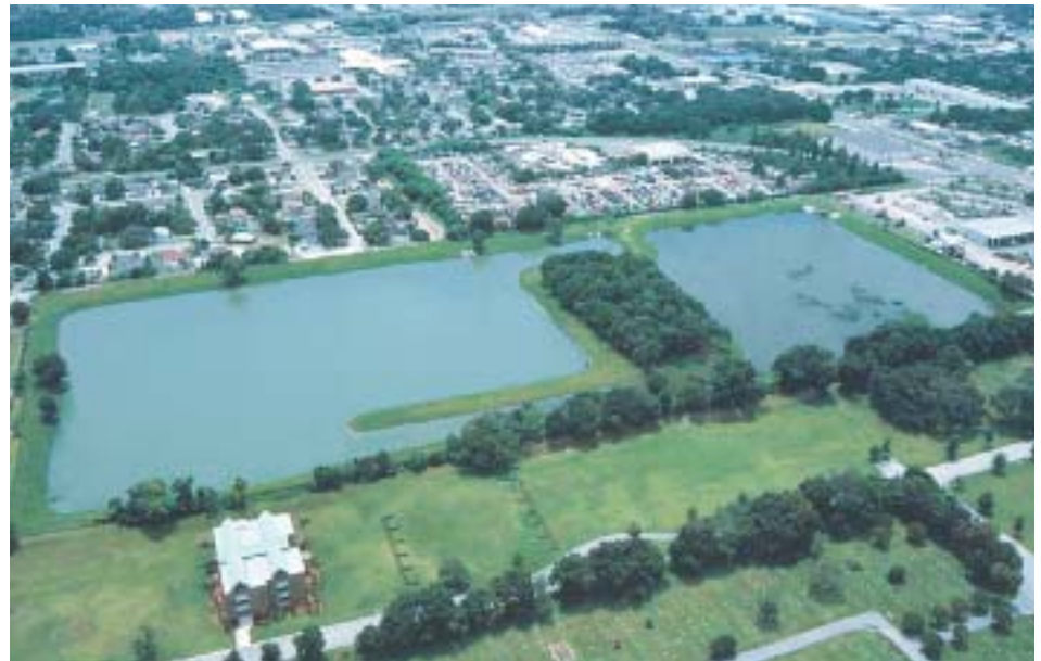
A consent decree established the first formal TMDLs in Florida in 1999. Solutions will involve short and long term projects. This wet detention pond provides both physical and biological treatment of stormwater.
