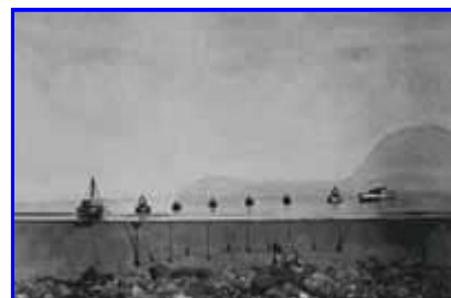
Wiredrag diagram. The basic principle is to drag a wire attached to two vessels. If the wire encounters an obstruction it will come taut and form a "V"
